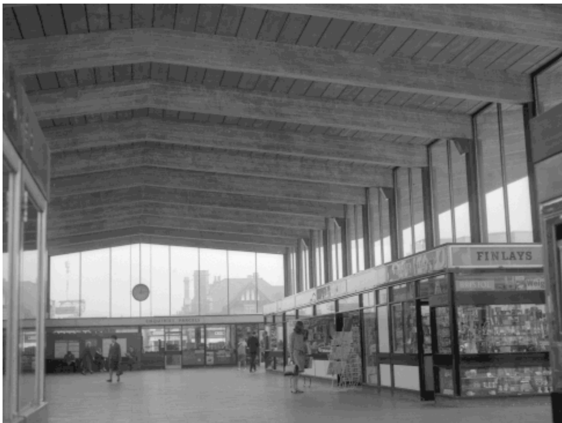
Figure 6: An internal view of Barking Station, around 1961
