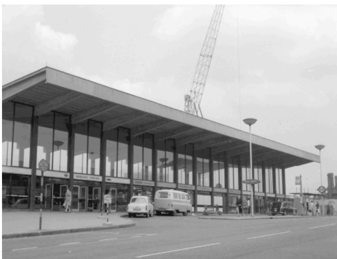
Figure 4: Barking Station shortly after completion in 1961
